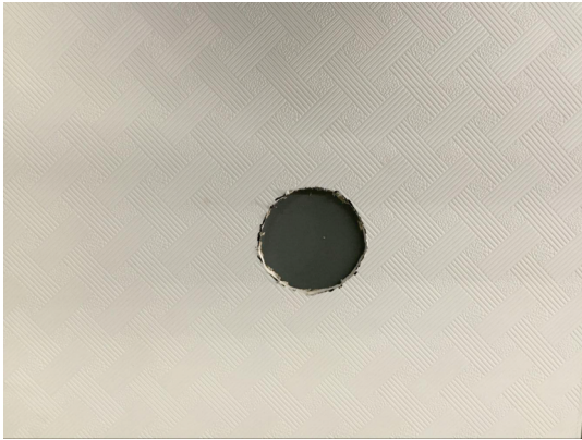
1. Drill a hole of \phi 95-105MM in the ceiling (FIG.1)
